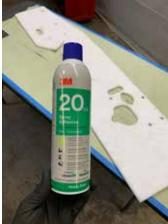
**Step 6**: White layer has previously been dry fit, so proceed with spraying aerosol adhesive on top of boom mat layer AND back of white layer for final installation. Follow aerosol directions for proper tack time.
